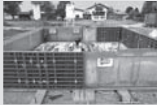
Wall Formwork
