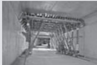
Tunnel Formwork
