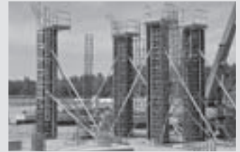
Column Formwork
