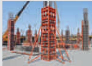
Column Formwork
