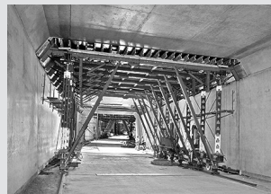
Tunnel formwork
