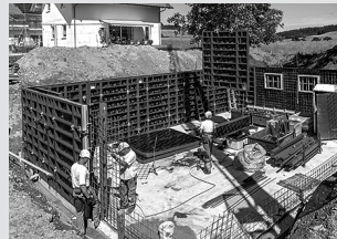
Wall formwork
