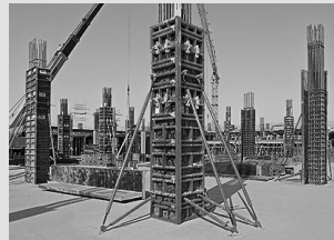
Column formwork
