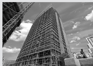
Working scaffolds façade
