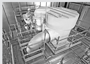
Working scaffolds industry
